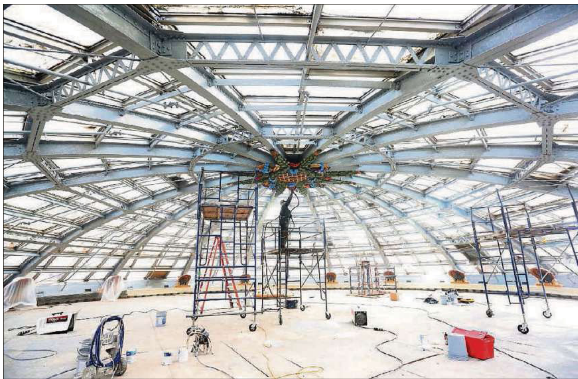
Since the Dayton Arcade opened in 1904, few people have had an up-close view of the top of the dome. A temporary wood deck has been constructed for renovation.
